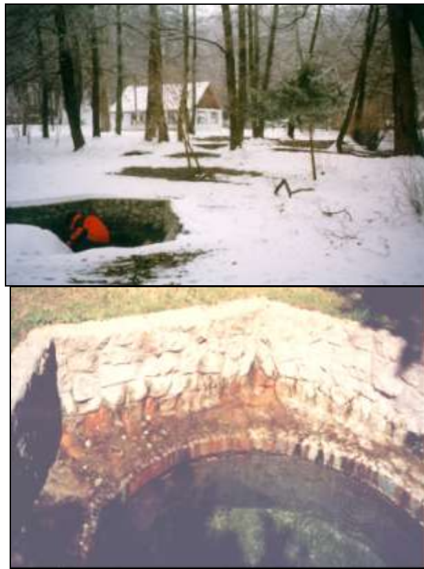
Fig. 4.3.3-4.3.4 Spring engaged for ecological purpose, Kács [Original, 1998, 2000]
