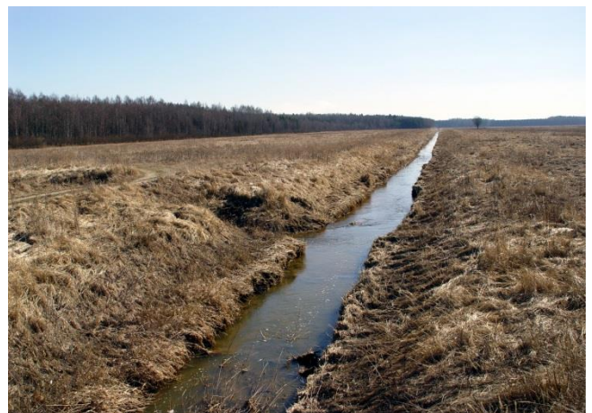
Figure 2. The channelized Slampe River, straightened in the 1970's draining the floodplain with abandoned grassland, photo taken in 2004 before the restoration activities. Photo: G. Pāvils
